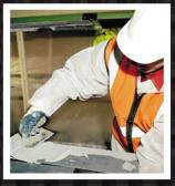
Composite fiber technology provides solutions for strengthening floors, walls, beams, columns and other structural elements suffering from deterioration, additional loads or excessive deflection. A need to increase the load capability of structures can arise from damage to structural elements, construction or design defects, alteration of design regulations, or change of use.
